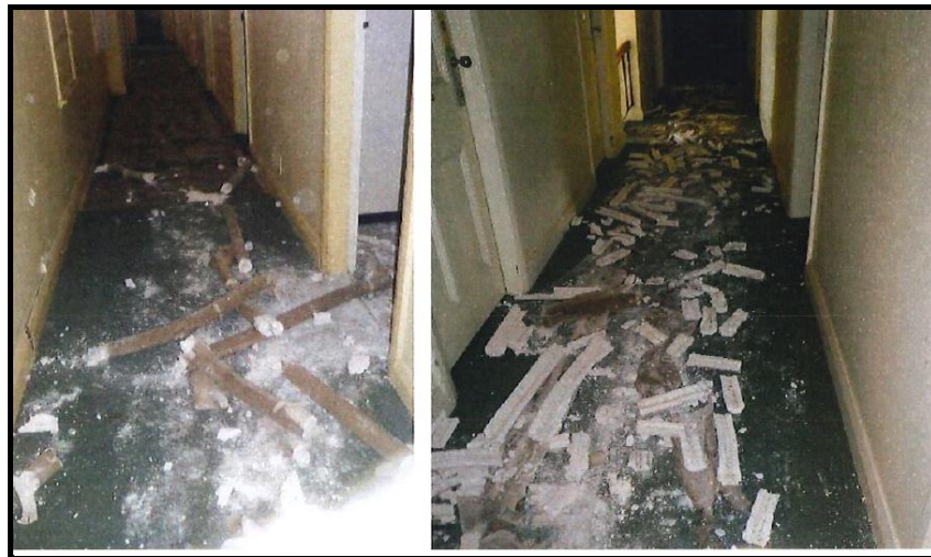
Figure 12: Corridor with asbestos lagging (Source: Asbestos Removal Options Report, Envirowest Consulting Pty Ltd June 2018)
